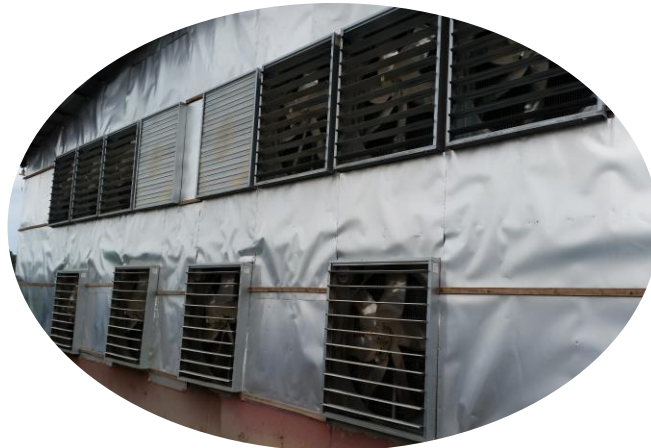
Efficient ventilation system
