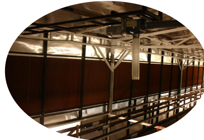
Air-conditioned system with air-conditioned wall
